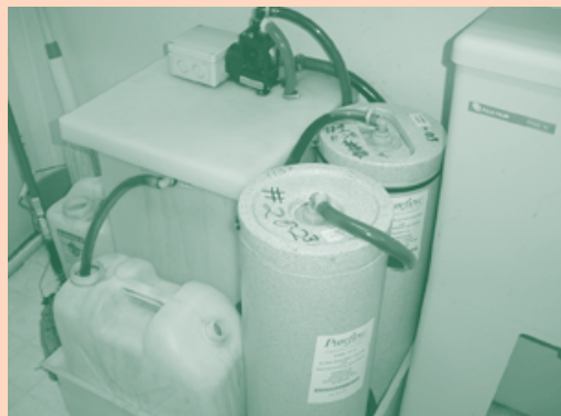
Photographic waste fluid treatment systems, like this one with dual cartridges to filter out silver, need to be regularly serviced and properly maintained to effectively remove silver before fluids can be safely sent to the sanitary sewer.
