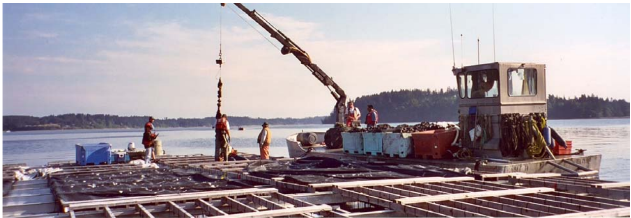
Figure A-4: Barge with Crane
