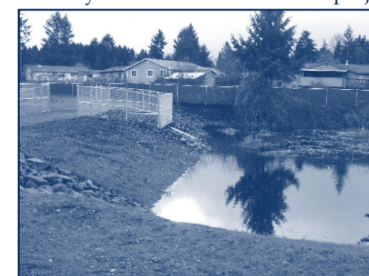
The Mallard Pond project will help protect Little McAllister Creek.
