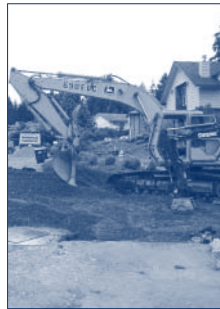
Construction at Lakemont and 49th.
