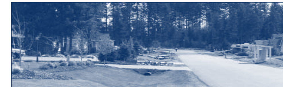
A well-maintained swale in the Countrywood Park neighborhood.
