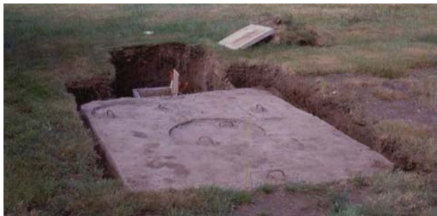
Exposed septic tank.
