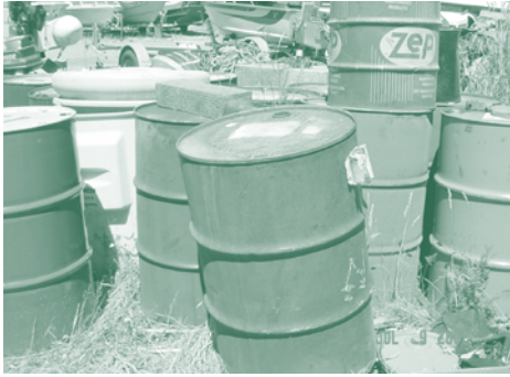
Storing full drums of hazardous waste outdoors without secondary containment is a violation of the county ordinance.
